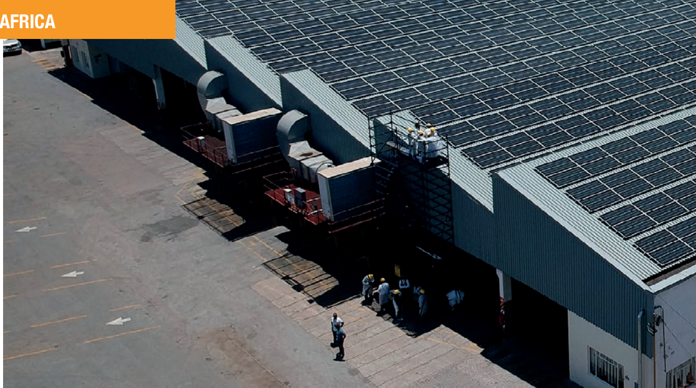
Figure 1: 1MW solar plant installation on the rooftop (9000sqm) of Schweppes Zimbabwe Limited (SZL) Harare factory 8
