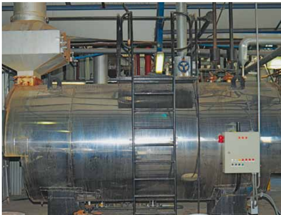
This boiler burns prune pits to make steam for processing
